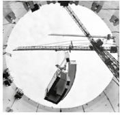
Cover photo: Installation of the reactor at Power Unit No. 5 of the Zaporizhzhia NPP, 1988. Photo No. 9366(14) from the collection of the State Archive of Zaporizhzhia Oblast.
