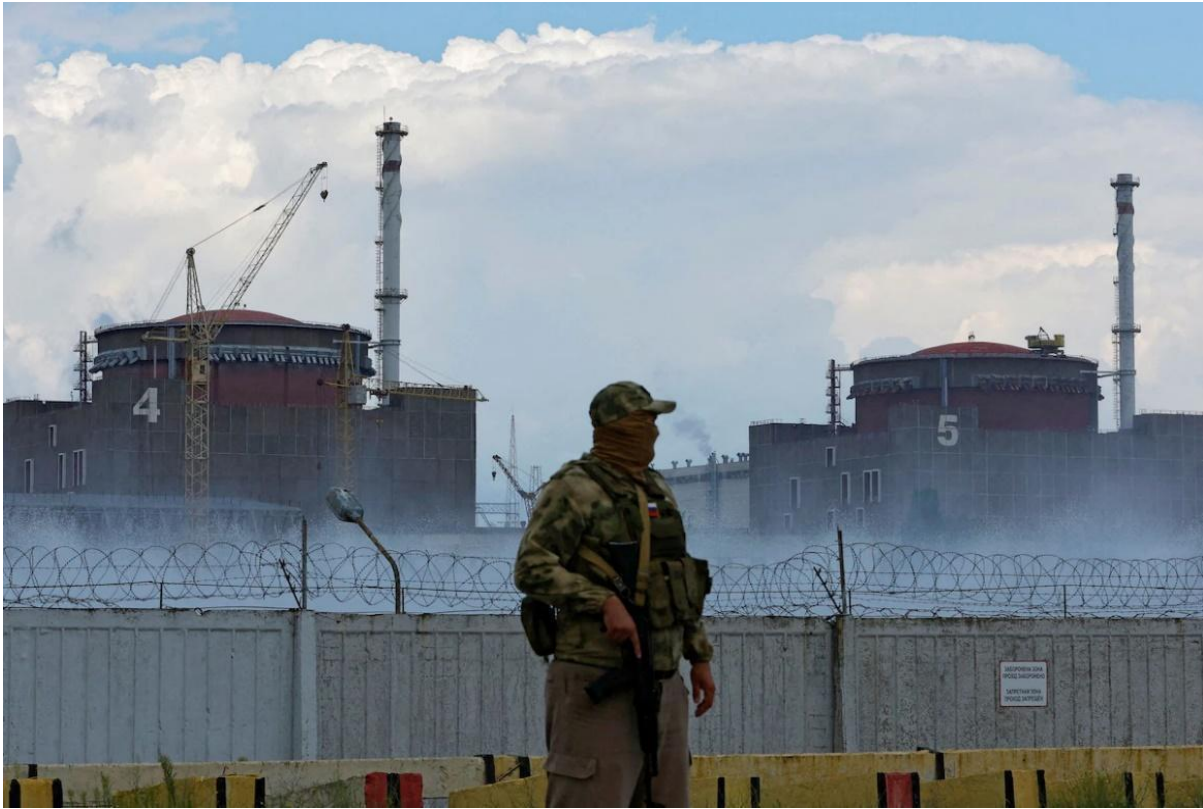
Figure 1. Russian military serviceman stands guard near the Zaporizhzhia nuclear power plant, August 4, 2023. (Alexander Ermochenko/Reuters)
